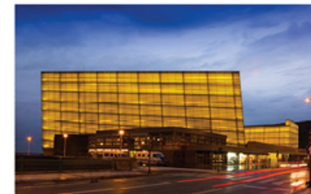
Kursaal Congress Centre and Auditorium
